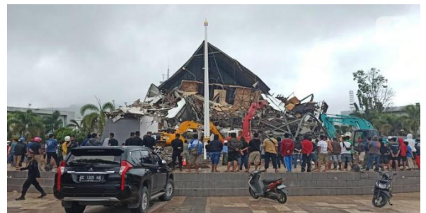
Governor office collapsed
